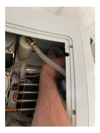
3. Slide the old filter off the filter housing and replace with the new filter.
